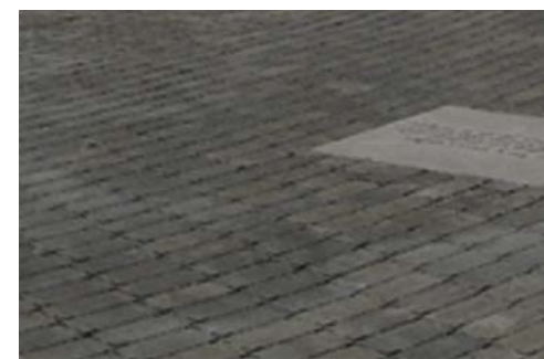
C GRAY BRICK PAVERS TO MATCH R.O.W. IMPROVEMENTS DESCRIPTION: PERMEABLE UNIT PAVERS COLOR: GRAY SUPPLIER: BORGERT SIZE: 5" x 10"
